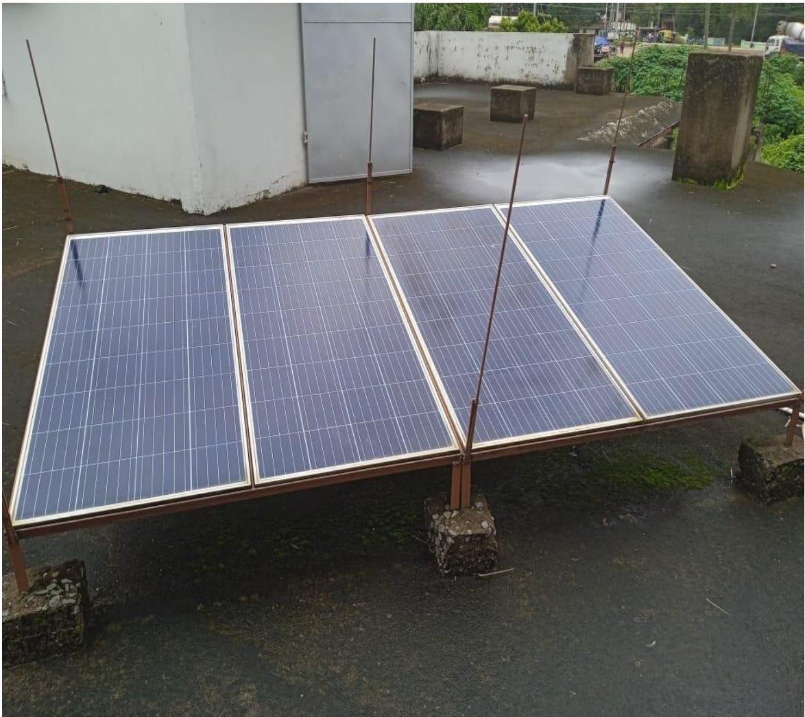
(Installation of Solar Panel)
